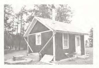
Figure 101. Deer Springs lookout cabin. Note the cistern at left and drains from the roof.
